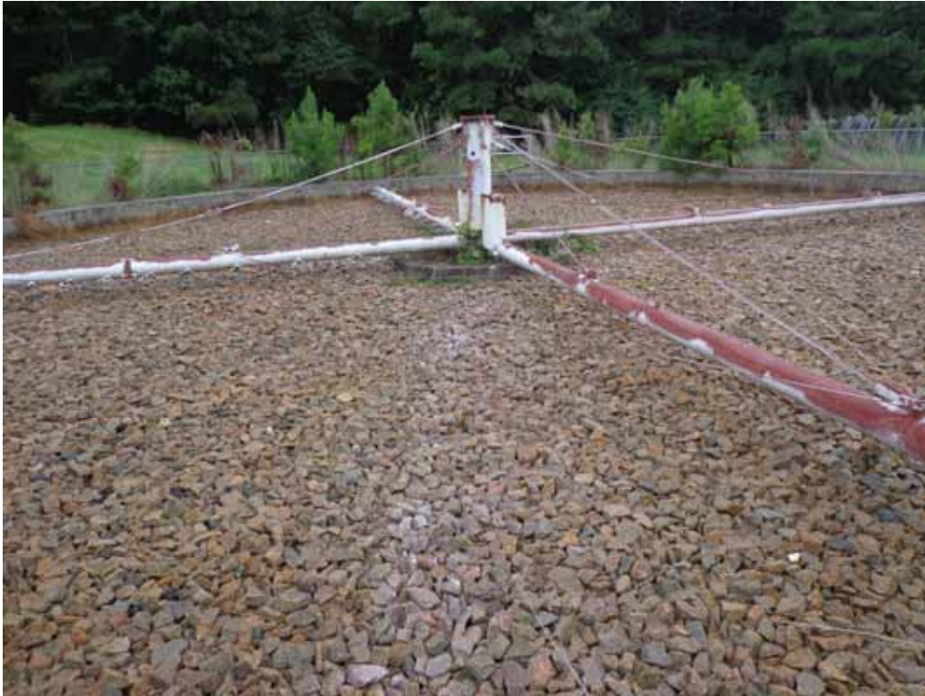
19. Trickling filter containment.
