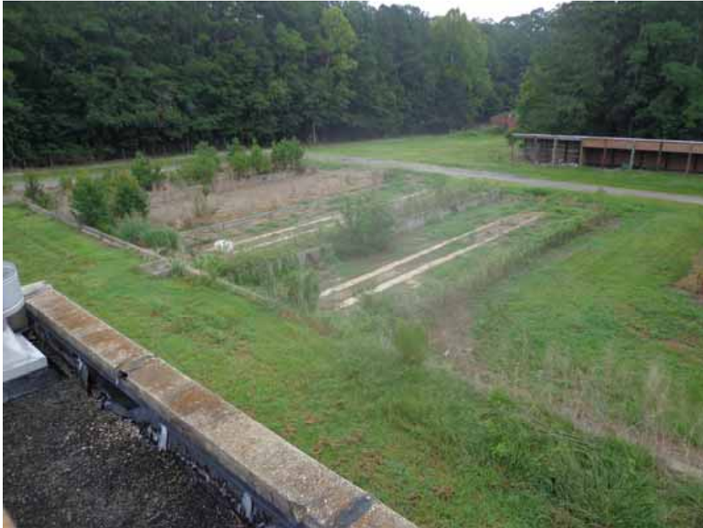
8. Slug drying pits.
