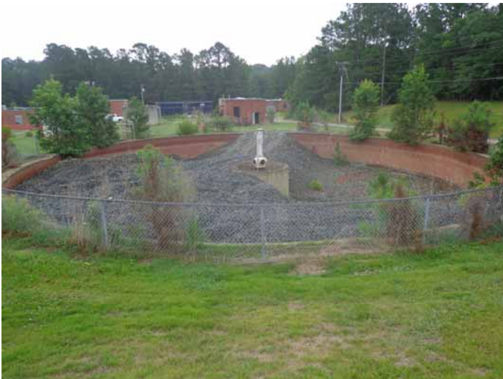
20. Secondary trickling filter containment.
