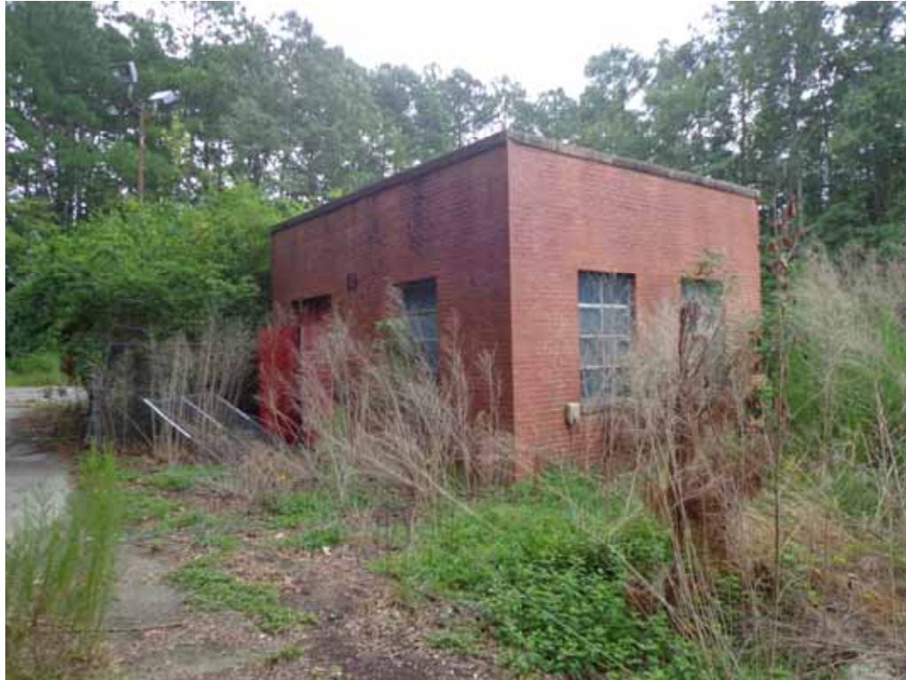
17. Plant pump station where influent came to the plant in its raw state.
