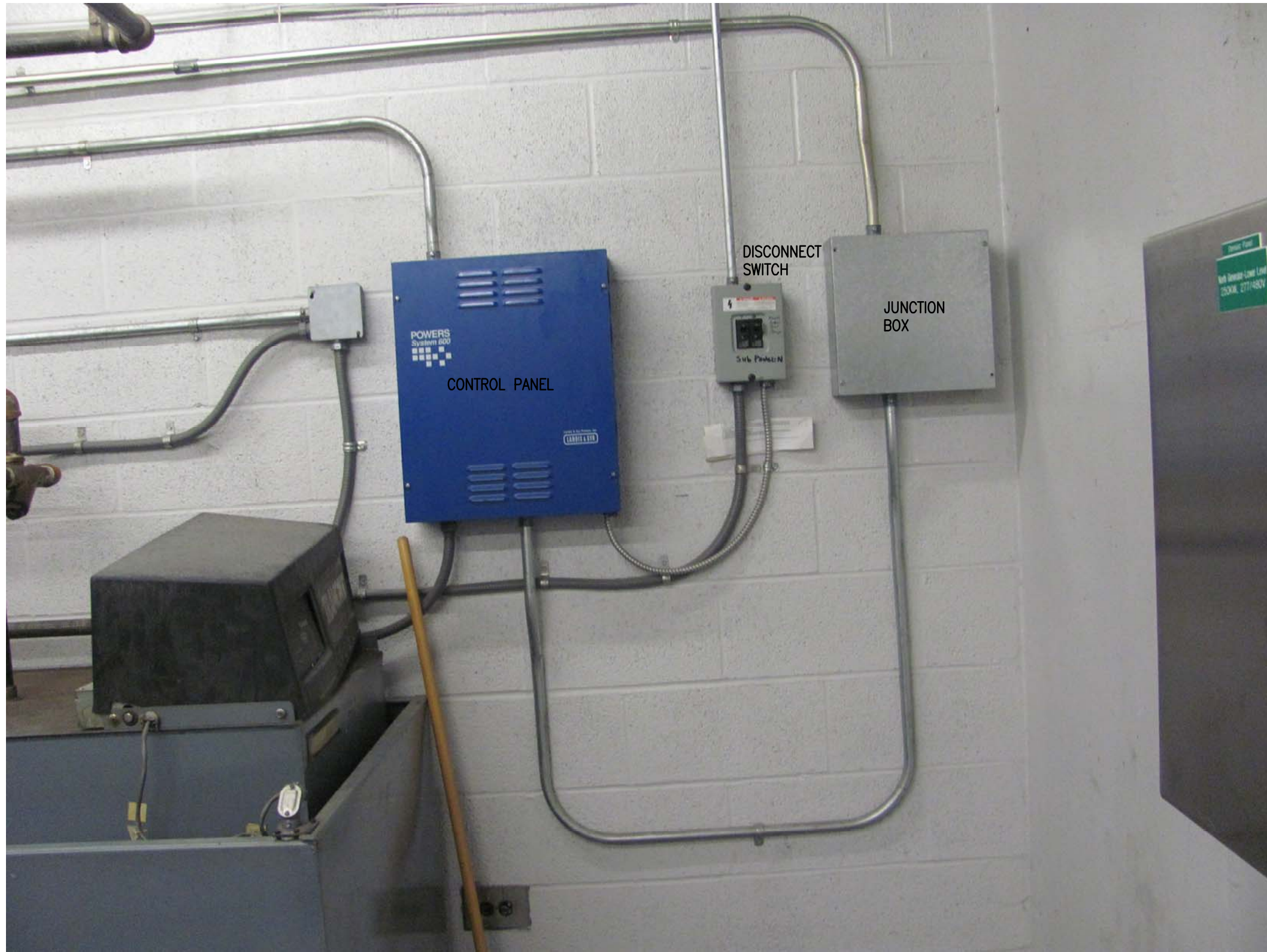
EXISTING FUEL CONTROL DEVICES PHOTO – NORTH GENERATOR ROOM NO SCALE
