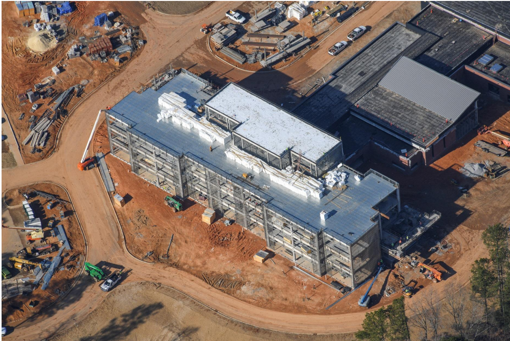
December 30, 2017 Roofing in progress and the 3-story classroom wing is topped out with metal deck, awaiting lightweight concrete.
