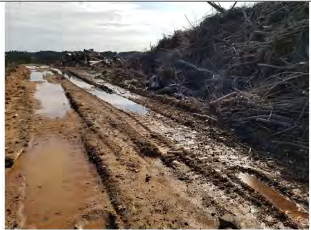
Figure 16: Water ponding ontop of inactive C&DLF.
