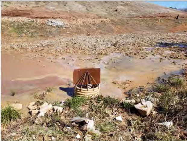
Figure 7: Basin 3 with leachate from LR3 and LR4 flowing into it.
