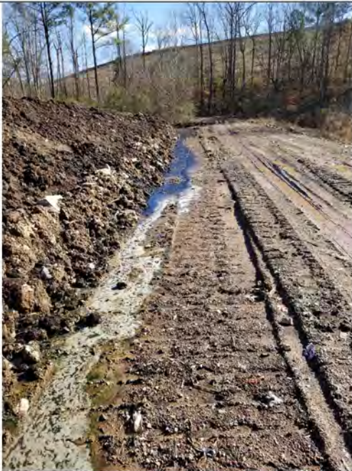
Figure 7: Leachate Release 5 along the southern edge of the Northwest Compost Area.
