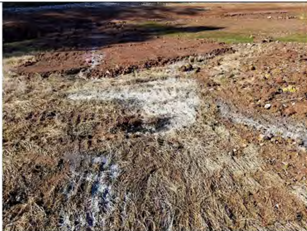
Figure 3: Leachate Release 2 on the northwest slope of the closed CDLF. This is the same location where a seep had been noted in the October 29, 2020 inspection.
