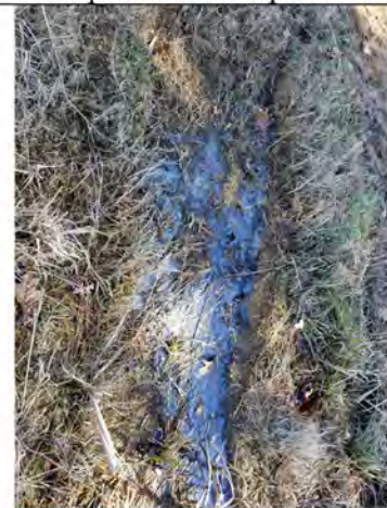
Figure 4: Leachate Release 3 on the southern slope of the closed CDLF.
