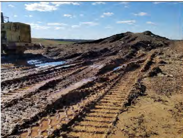
Figure 15: Water impounding over waste (CDLF) and around waste (mulch).
