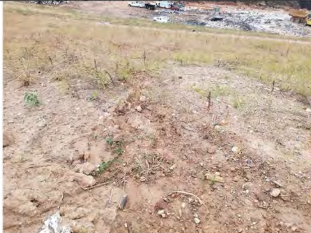
Small erosion rill on CDLF.
