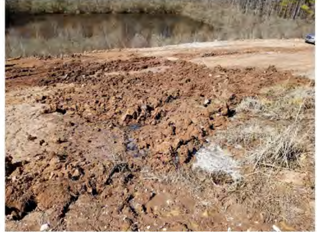
Figure 4: LR2 dammed by earthen berm.
