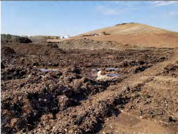
Figure 17: Water ponding in and around compost operational area.
