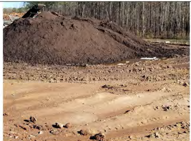
Figure 16: Water ponding in compost operation area.
