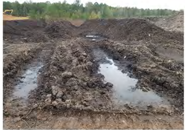
Water ponding in compost operational area.
