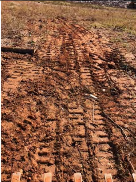
Erosion rill repair.
