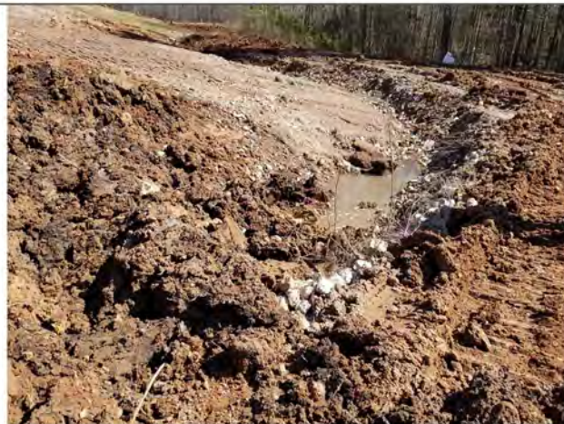
Figure 10: LR4 flowing into ditch with soil plug.
