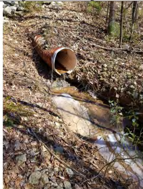
Figure 8: Outflow of Basin 3 contaminated with leachate from LR3 and LR4.
