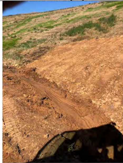
Repair to ditch along CLDF edge of waste that had been retaining water.
