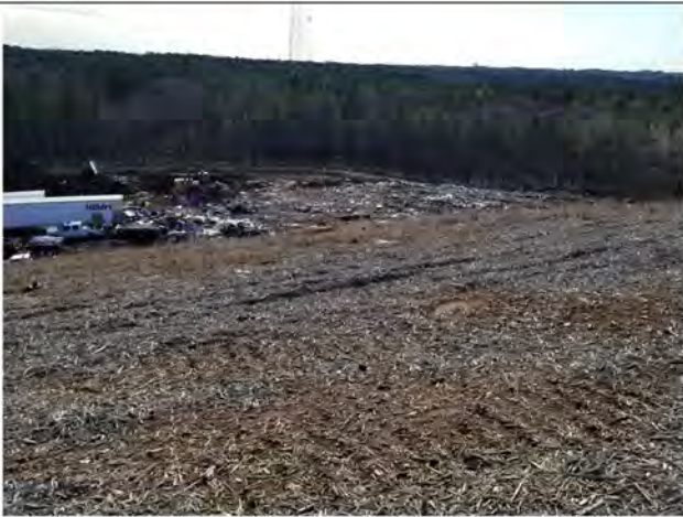
Figure 21: Working face of C&DLF appears to be larger than half acre.
