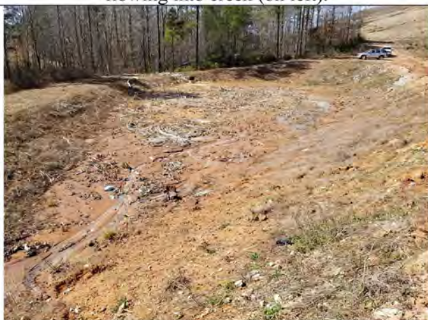
Figure 11: LR4 flowing through the soil plug into Basin 3.
