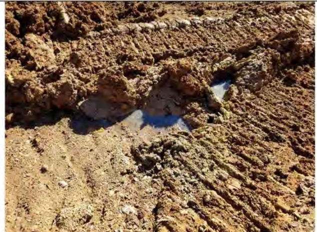
Figure 6: Leachate Release 4 on the southern slope of the active CDLF. This area had been plugged, but it did not adequately resolve the flow of leachate.
