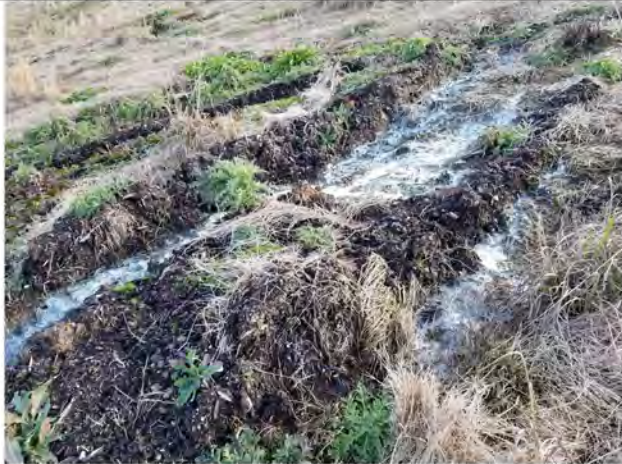
Figure 1: Leachate Release 1 on north slope of closed CDLF.
