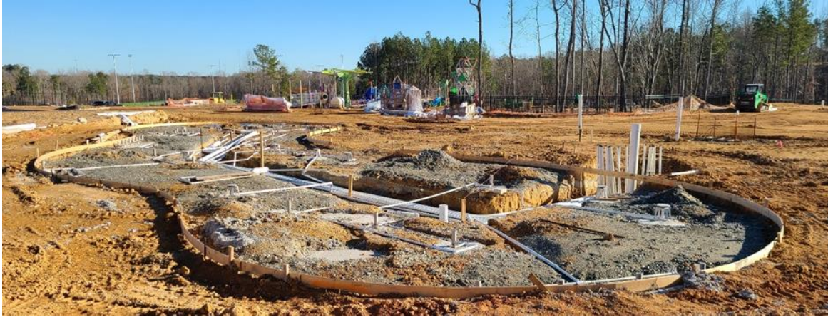
FIGURE 7: CONSTRUCTION OF SPLASHLANTIS WATER PLAY PARK FOR PLEASANT PARK IN THE TOWN OF APEX.
