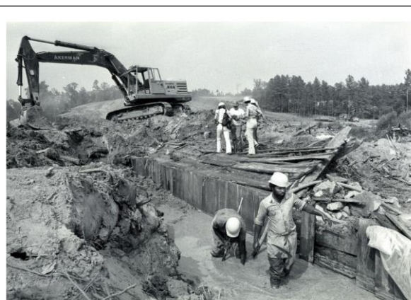
Figure 1. Construction of the Falls Lake Dam, photograph courtesy of the US Army Corps of Engineers as cited by the Wake Forest Historical Museum.
