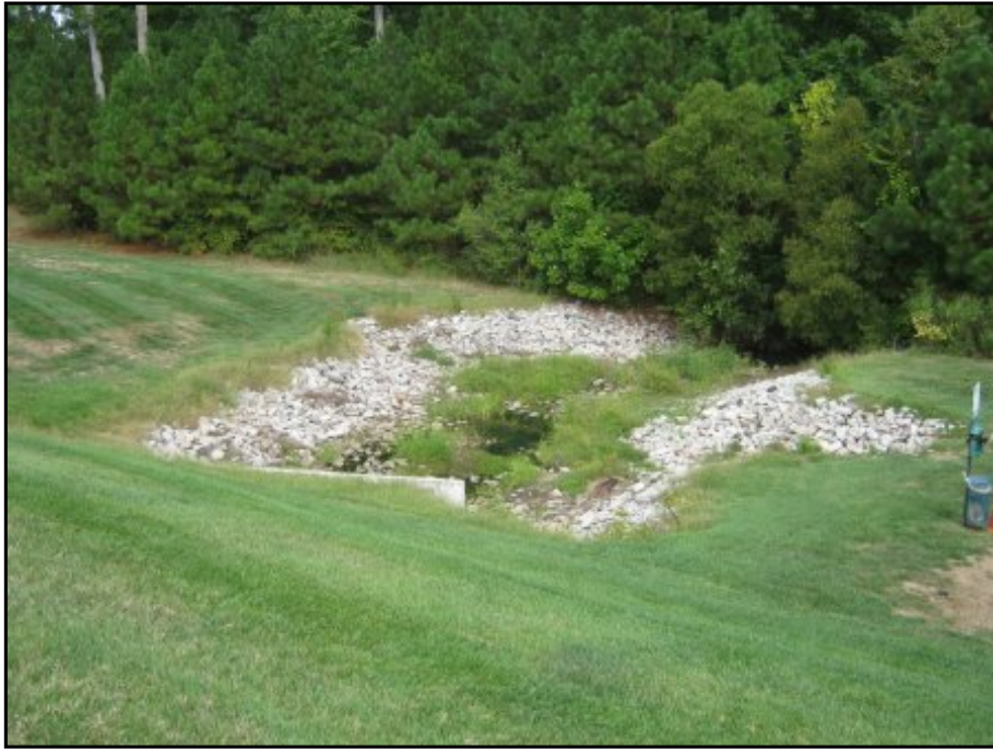
View of stormwater culvert adjacent to the south of the Property.
