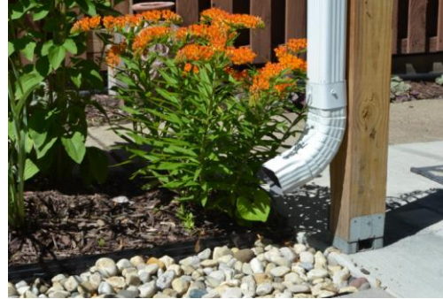
Roof drain disconnection
