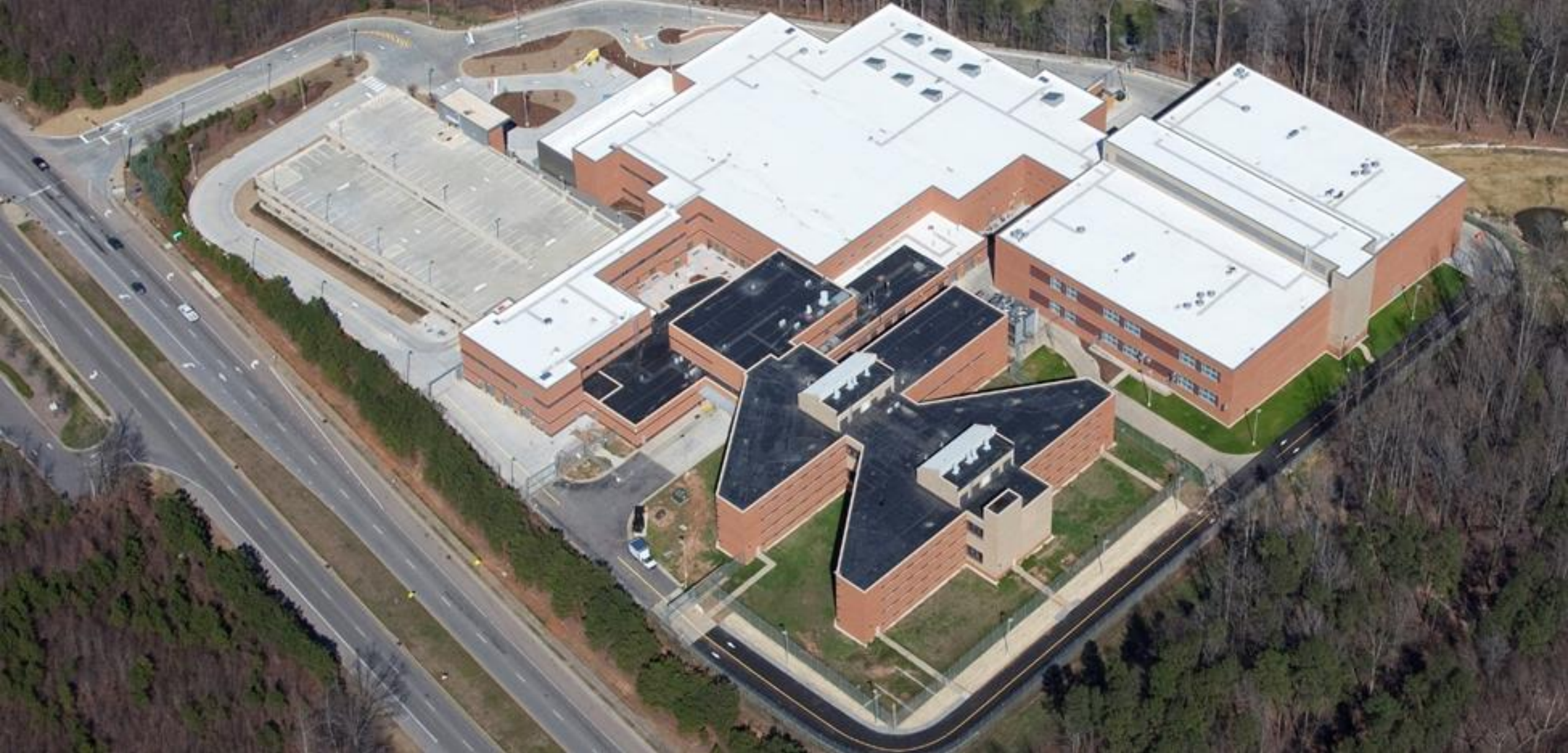
Existing Wake County Detention Center - 3301 Hammond Road
