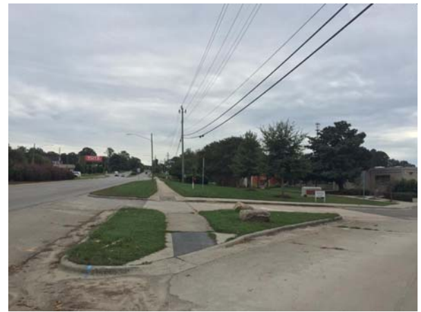
View of subject property looking south along South Wilmington Street
