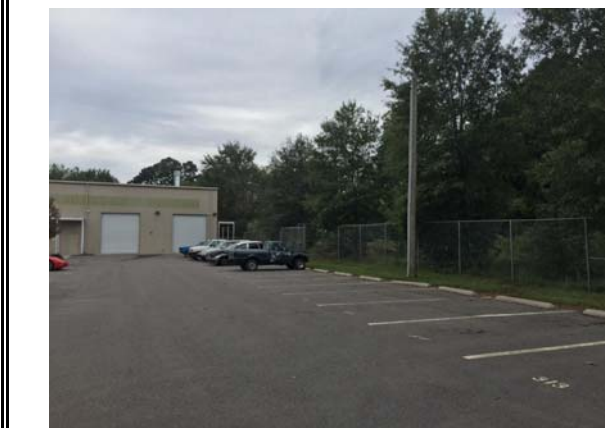
Interior view of subject property in vicinity of planned easement corridor
