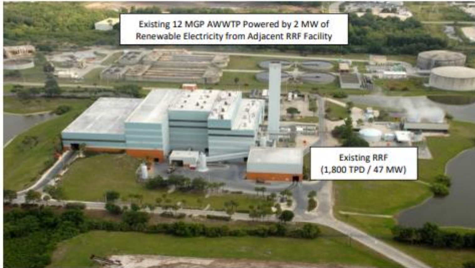
Figure 1. Hillsborough County, Florida RRF Facility provides 2 MW of Renewable Electricity to 12 MGD AWWTP and other adjacent Public Works
