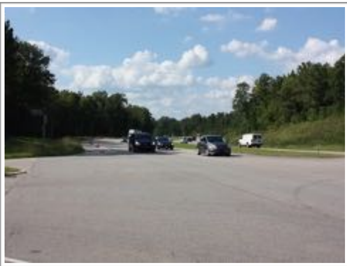
View North Along Davis Drive from Little Dr.
