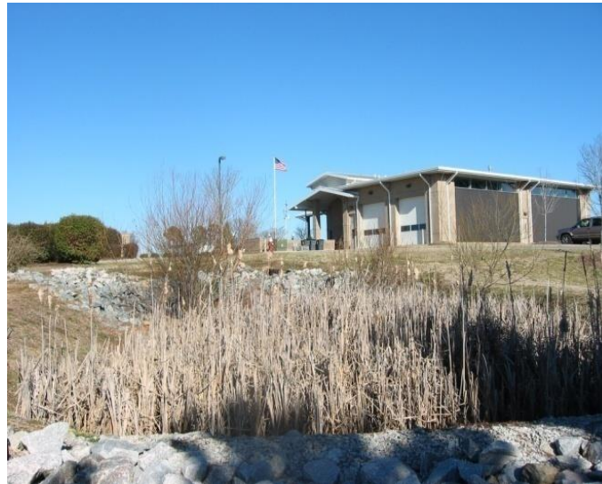
Willow Springs Fire Station Rain Garden
