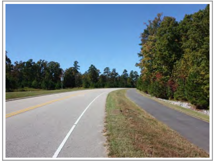
Little Dr. View West Along Frontage
