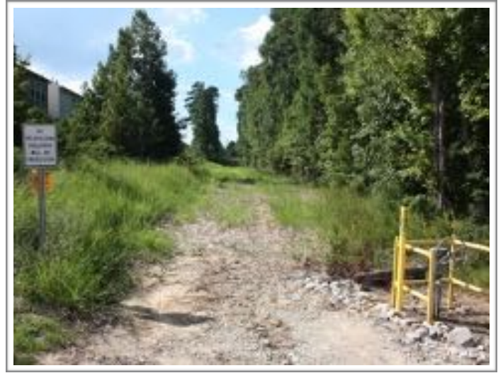
Interior Utility Access
