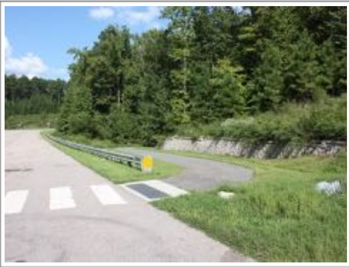
Greenway Entrance Near Intersection
